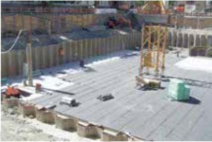
The new construction of the Vicentius Area at Laubenhof in Konstanz aims to fulfill the desire for modern living in the city center. As an additional safety measure, our **wolfseal** FBV sealing membrane was installed beneath the floor slab.
